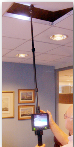
Inspecting the area above a suspended ceiling.
